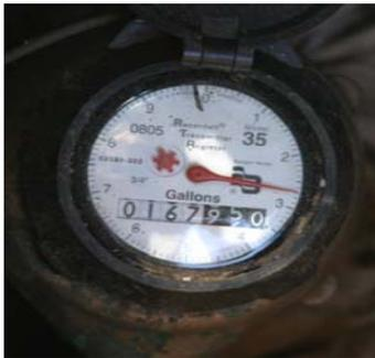
Step 3. Take the lid off the meter box and lift the protective cover. See “How to Read Your Water Meter” pamphlet for directions. **Watch the meter.** Your meter will have a red star wheel that is commonly called a “leak indicator.” If it is spinning, even very slowly, you have a leak. If it is not spinning, look at the red pointer and note the number it is pointing at.
