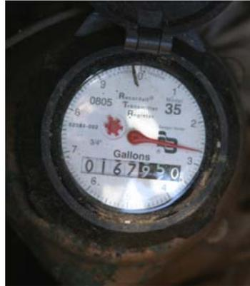
see a large dial, a small red star wheel and a set of numbers similar to a car's odometer. The large dial typically reads gallons. The small star wheel is used to detect leaks and minor usage. The odometer reads total gallons used. Read the odometer left to right, including the fixed zero on the far right.
